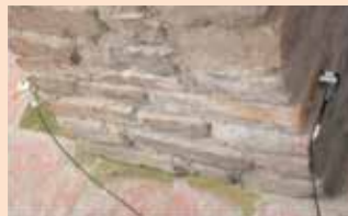
Image Ref. 3.14 Measurement of brick wall Source: Junji Kiyono
