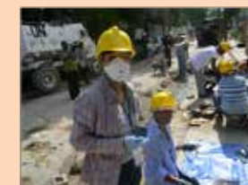
◀ Image Ref. 3.50, 3.51 Salvaging objects from damaged structures post earthquake in Haiti. The instructor highlighted the importance of documentation of each stage and recording as much information Source: Aparna Tandon
