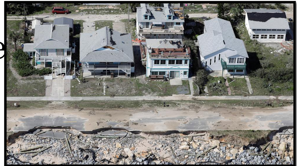
A1A wash out after Matthew
