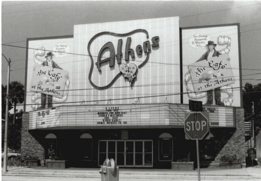
Athens Theatre, Deland – ca. 1970s Tax credit project to restore the historic appearance covered over
