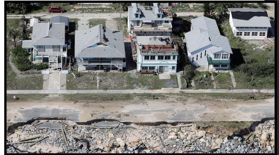
A1A wash out after Matthew
