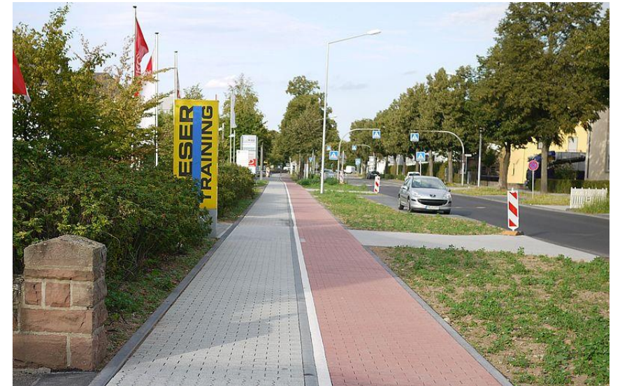
Example Sidewalk and Trail Project
